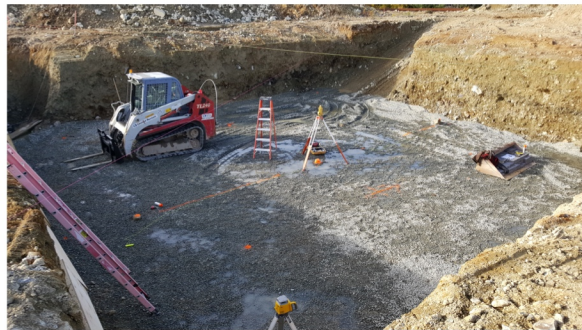
VOAR FM Tower Excavations, Oct. 30, 2017 Photo by: Brian Matthews
